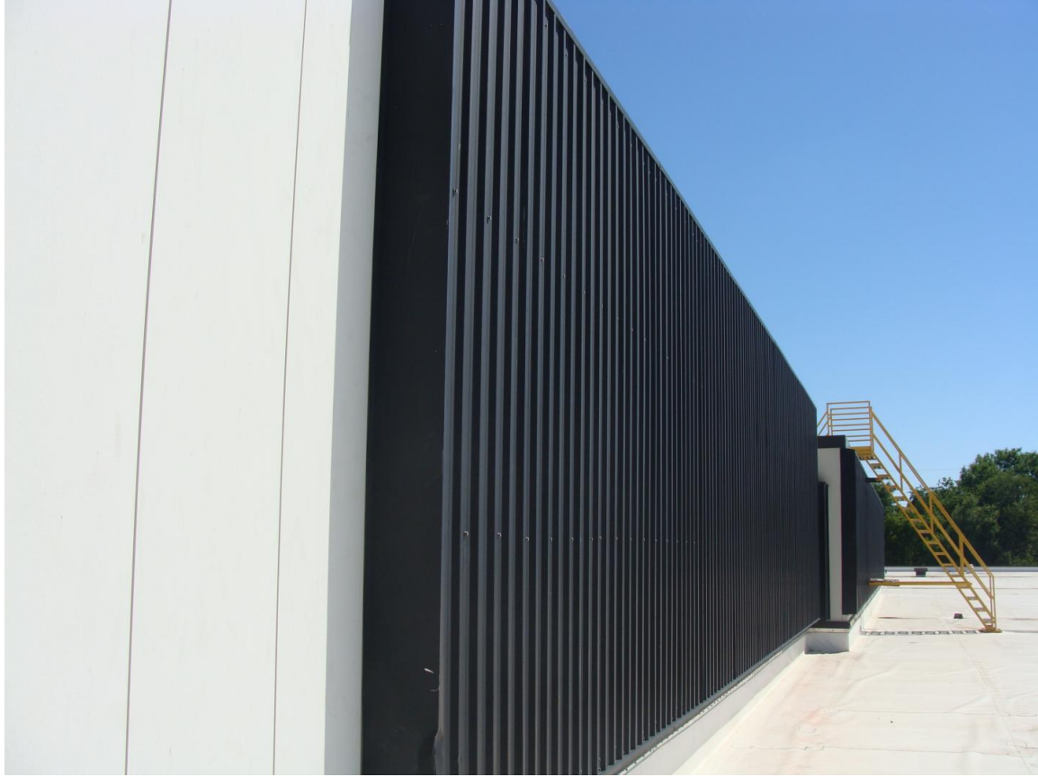
Figure 1.1.8: Solar wall installation at AVEDA Corporation Headquarters.
