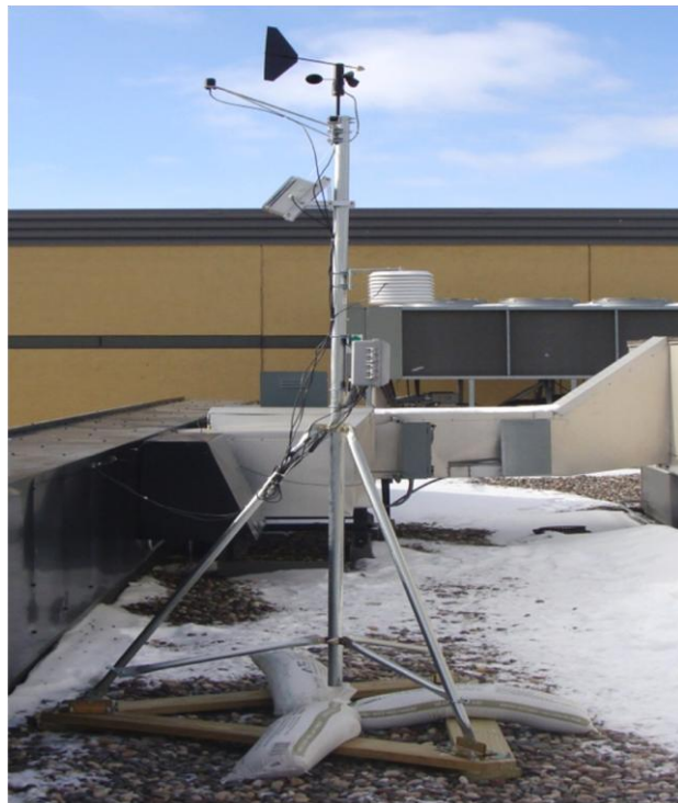
Figure 14: Completed 3 rd Precinct weather station.
