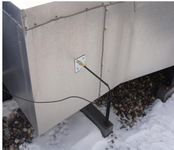
Figure 11: Close-up of first installed temperature sensor and mounting at 3 rd Precinct.
