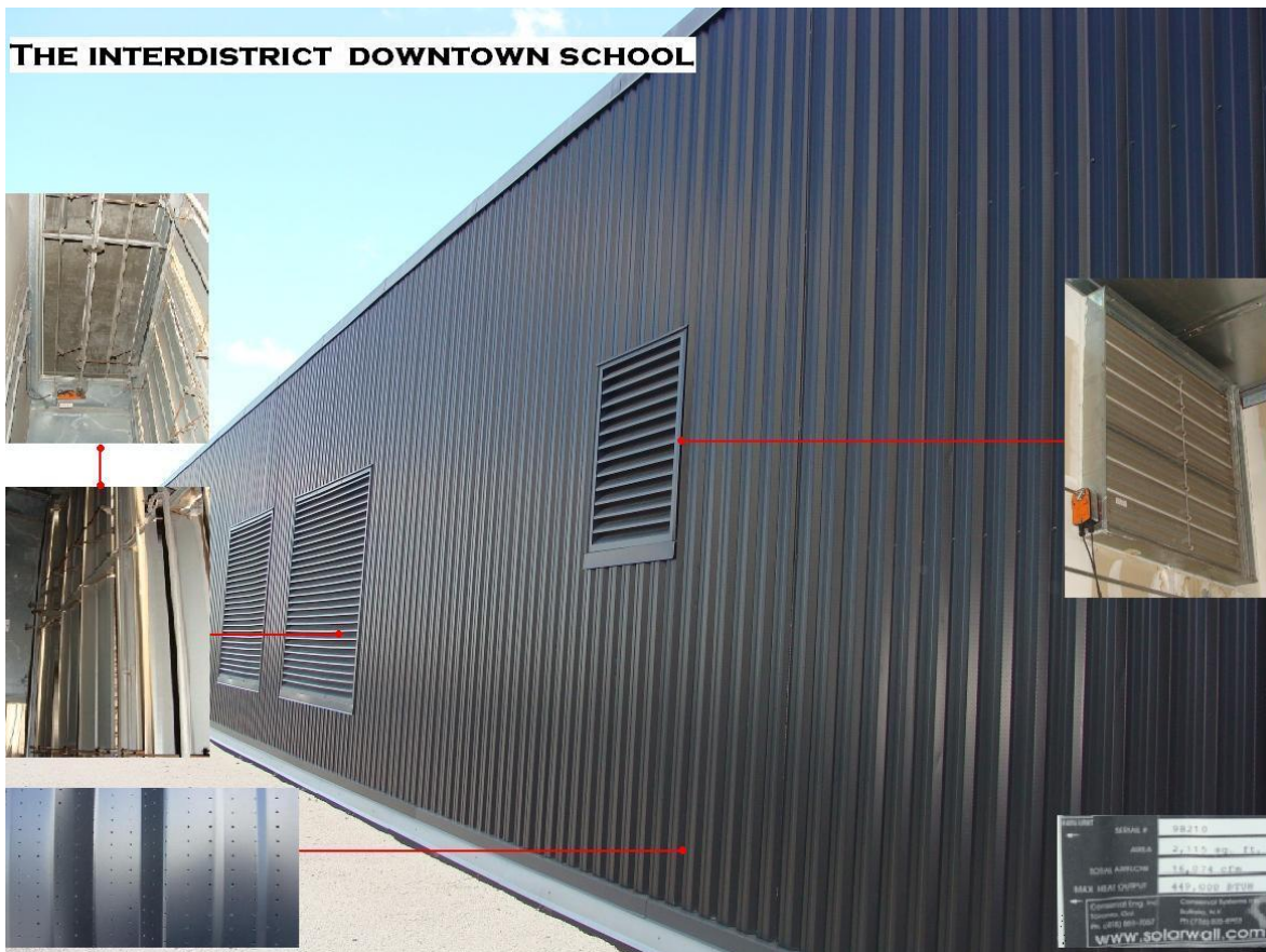
Figure 1.1.13: Breakdown of IDDS solar wall components.
