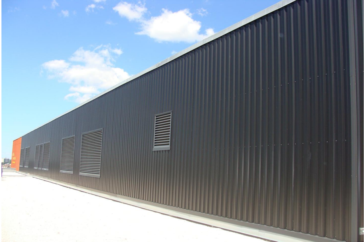
Figure 1.1.11: Solar wall installation at Interdistrict Downtown School.
