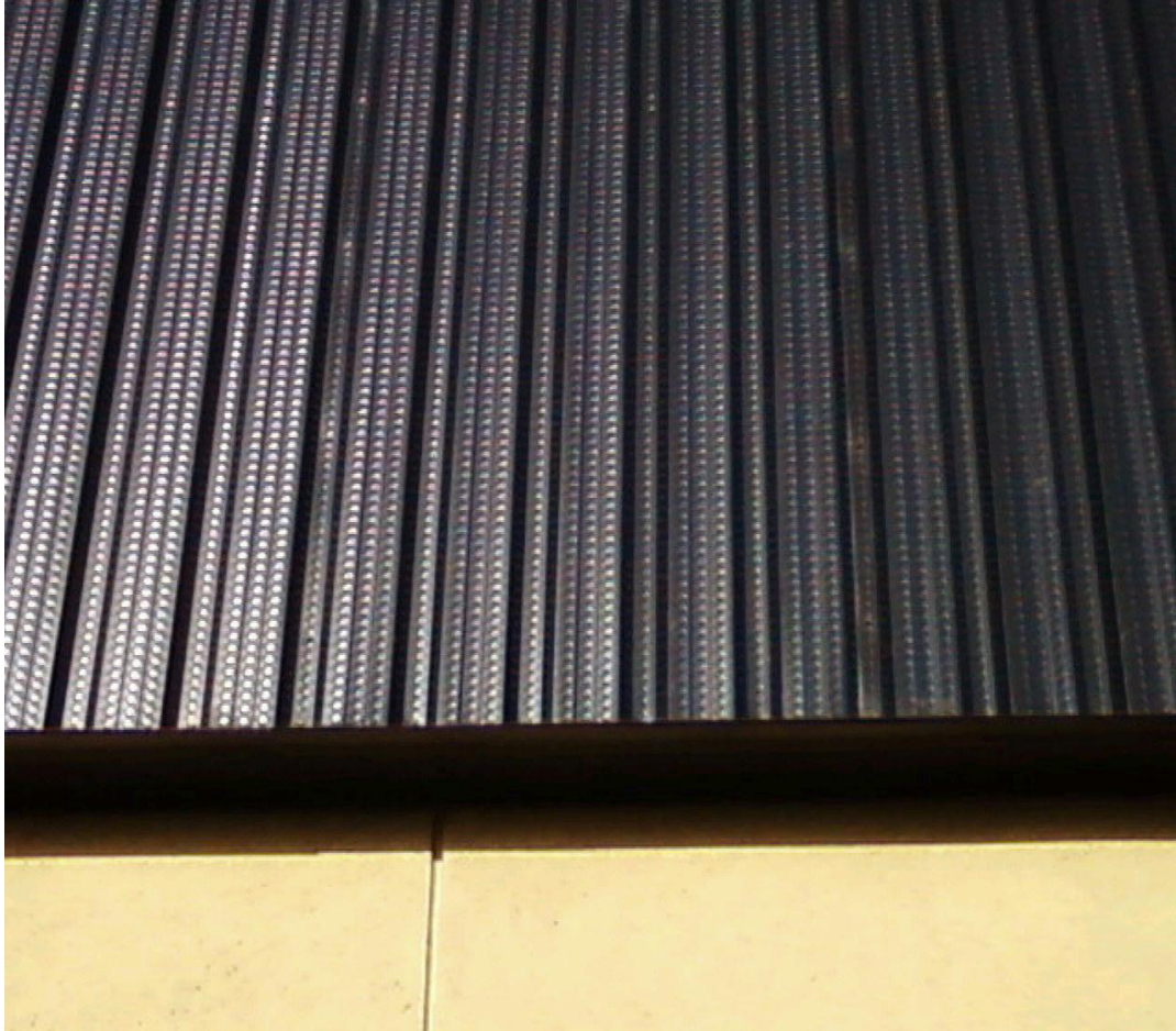
Figure 1.1.6: Close-up of 3 rd Precinct solar wall perforation patterns.
