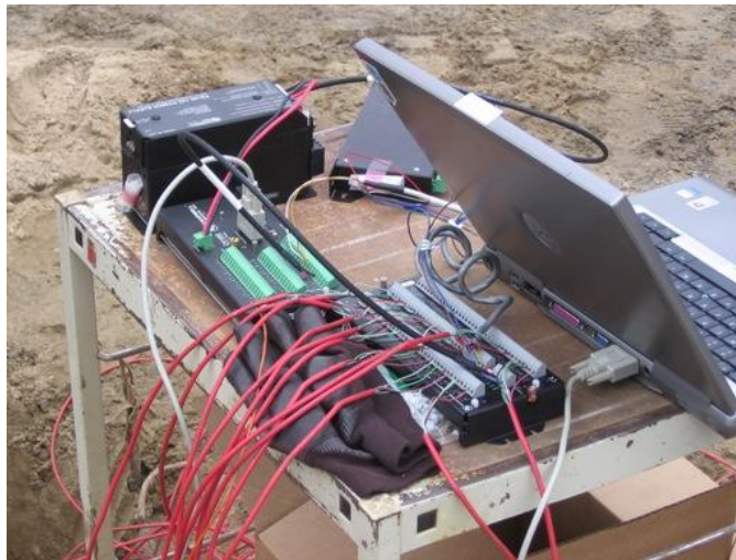
Figure 5. Data Collection Following Pile Driving
