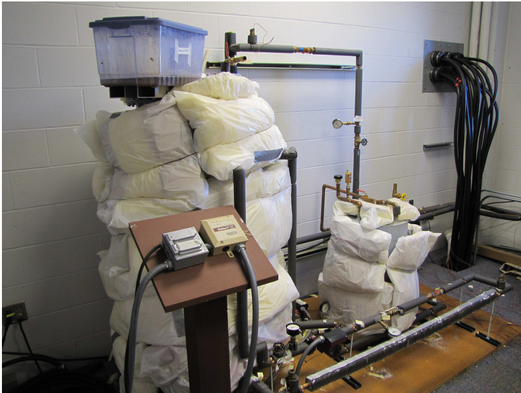
Figure 4: A Photograph of Transfer and Heating Loops
