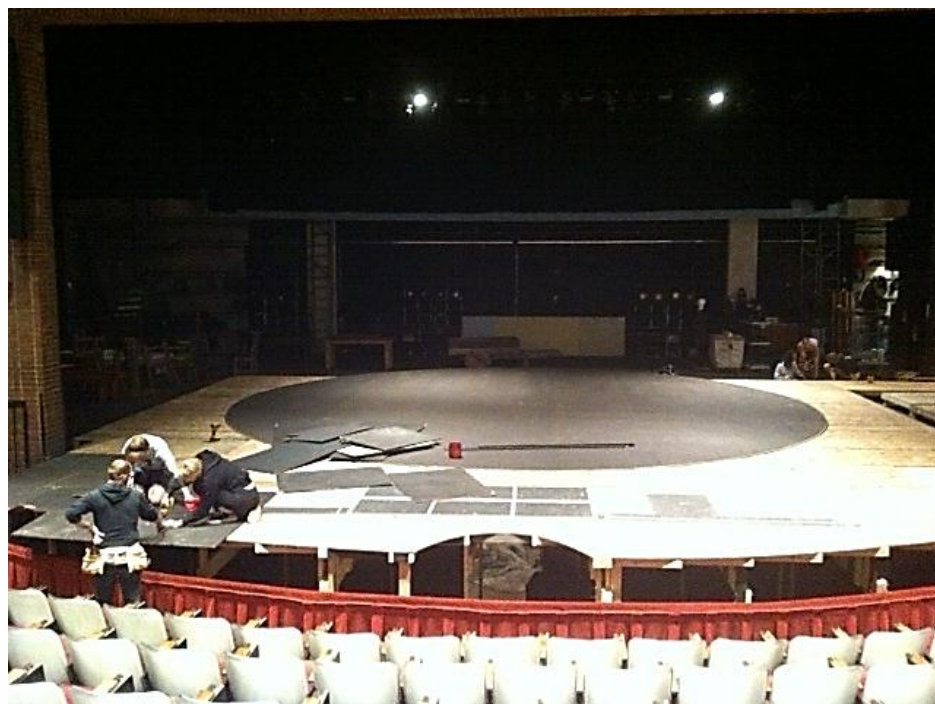
INSTALLATION OF SOUNBOARD ON ELEVATED FLOORING
