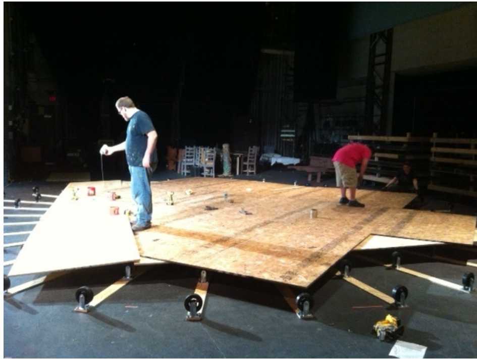
INSTALLATION OF PLYWOOD LAYERS
