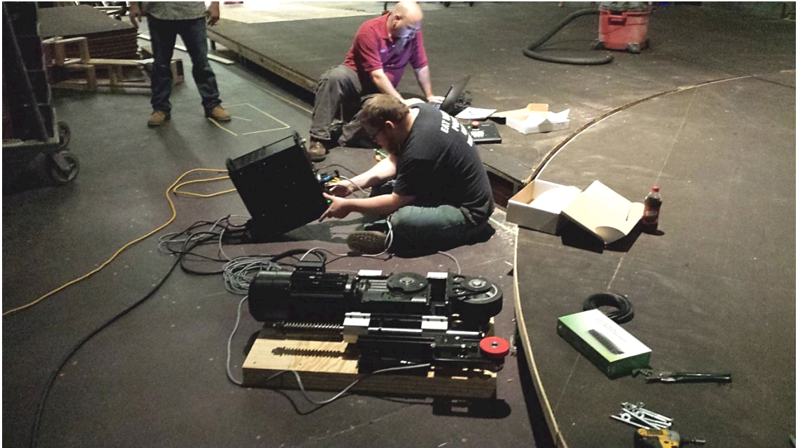
INSTALLATION OF AUTOMATION EQUIPMENT
