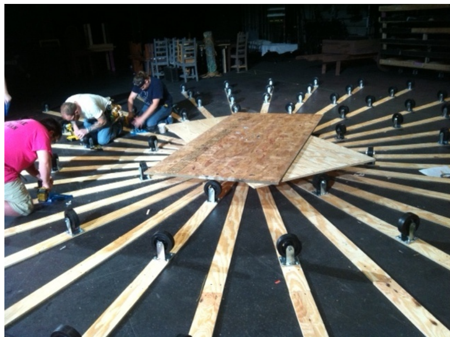
CASTER INSTALLATION WITH CENTER PIVOT PIECES
