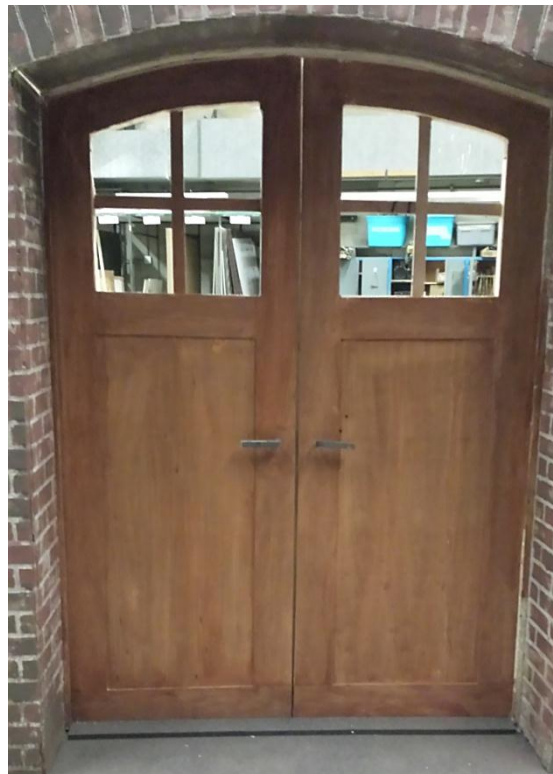
CUSTOM MADE HOLLOW WOODEN DOORS
