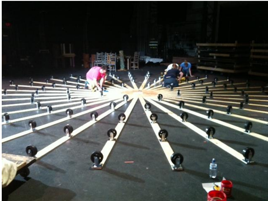
INSTALLING THE CASTERS
