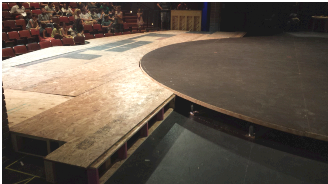
ELEVATED FLOORING PARTIALLY INSTALLED
