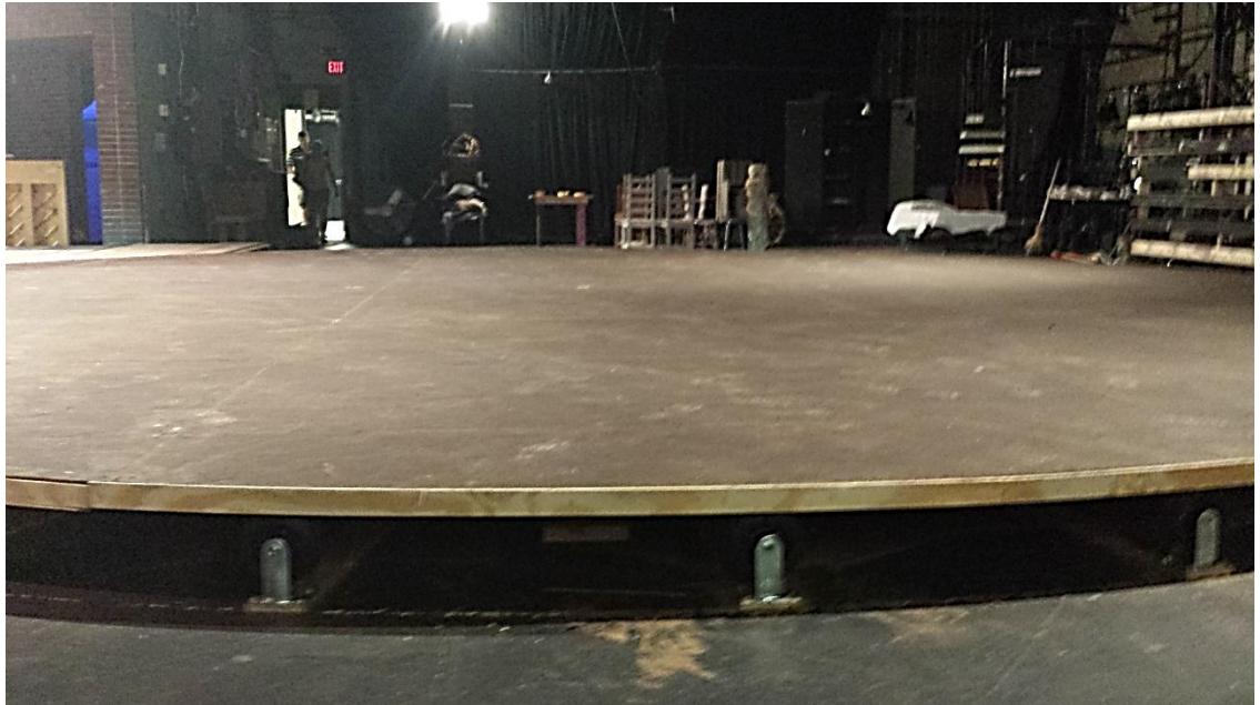
SOUNDBOARD AND OUTER TRIM ON REVOLVE INSTALLED
