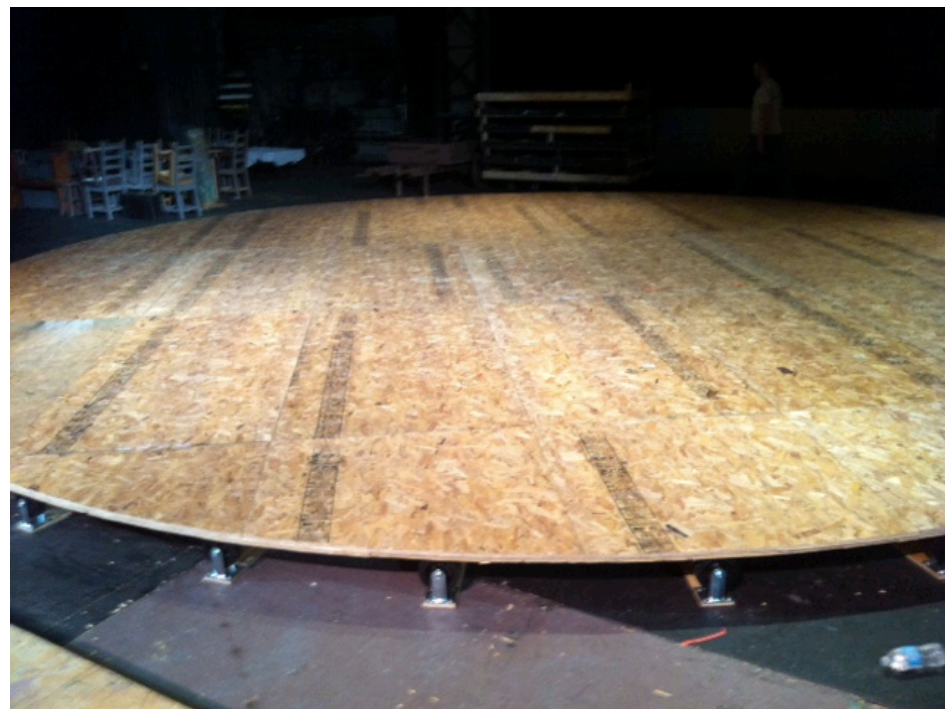
PLYWOOD REVOLVE COMPLETE
