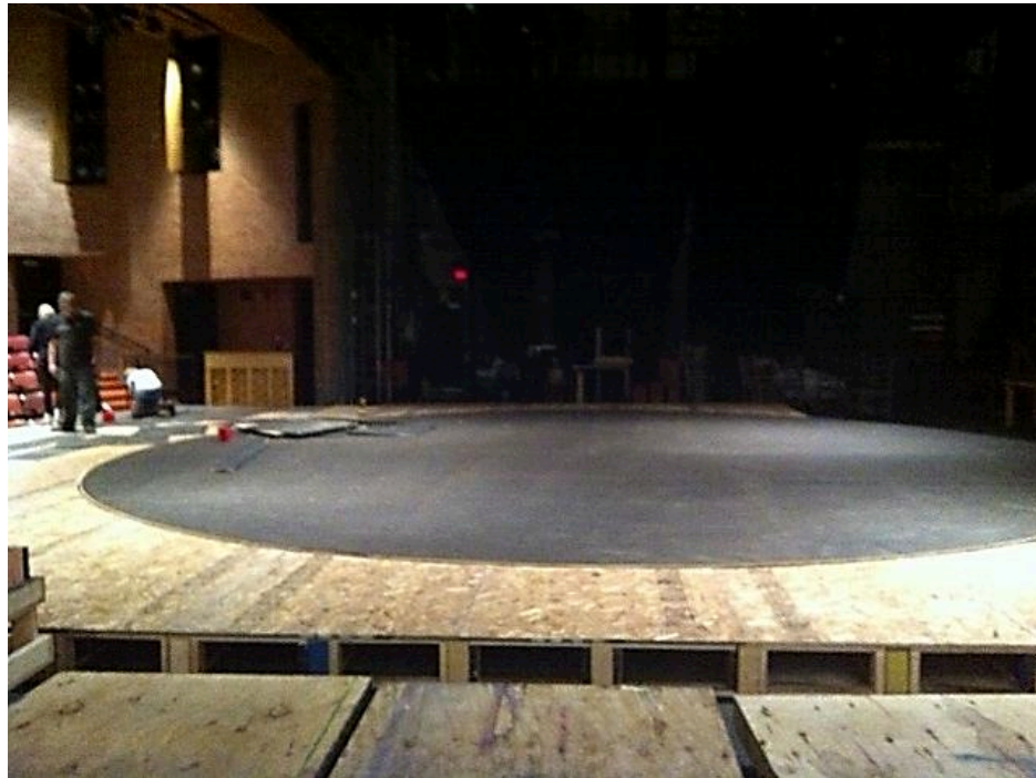
STUD WALL ELEVATED FLOORING COMPLETELY INSTALLED
