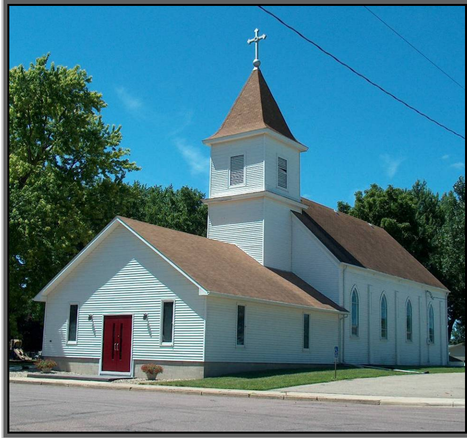
Figure 62: St. Joseph's Catholic Church, 2005 Vestibule added in 1975. (Photograph by author)
