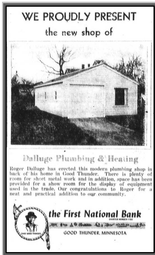
Figure 53: Dalluge Plumbing & Heating, 1951 (Image from the Good Thunder Herald , 6 December 1951.)
