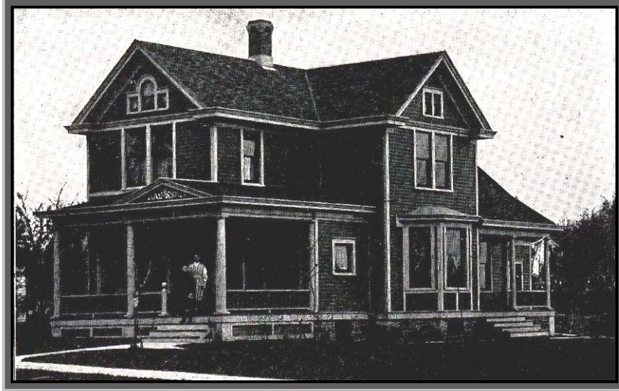
Figure 39: F. H. Morlock Residence, ca. 1910 Cross-gabled Queen Anne Victorian architecture. (Photograph from the collection of the Minnesota Historical Society)
