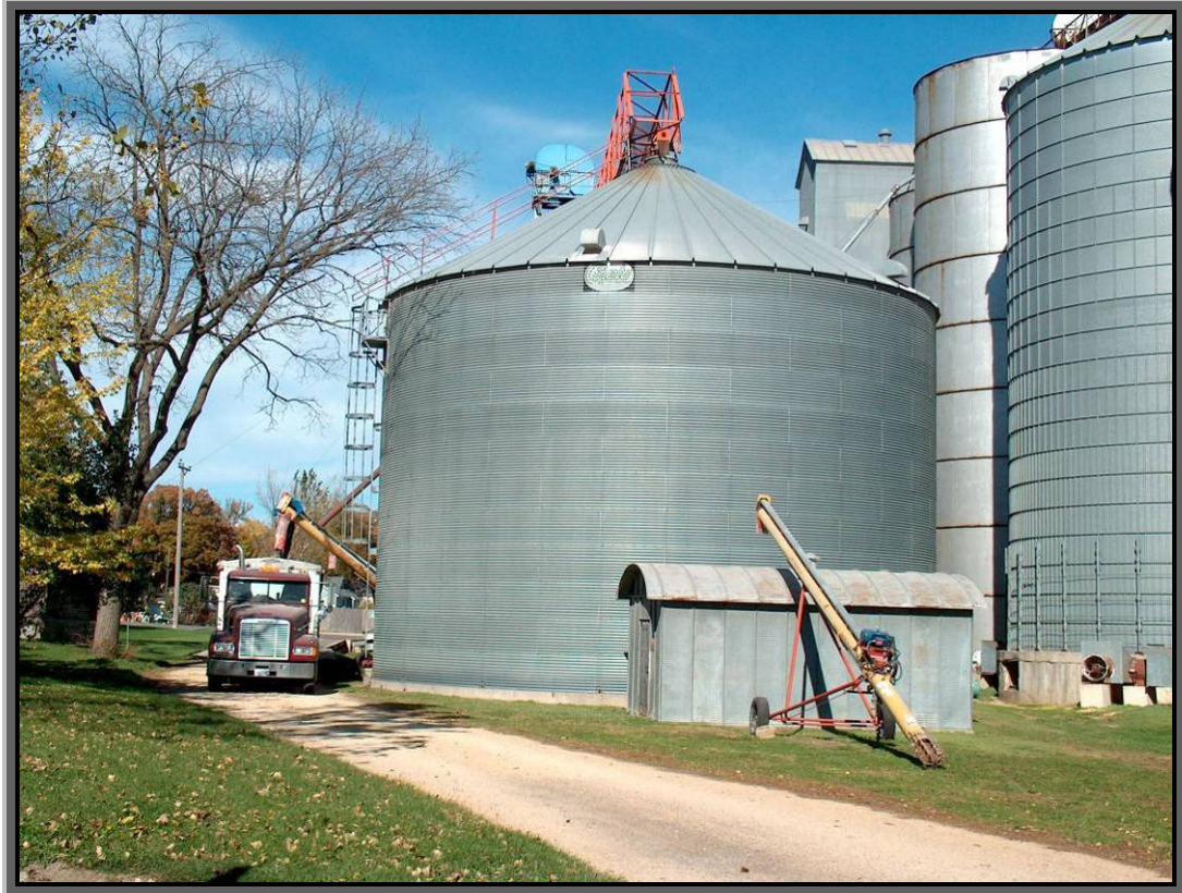
Figure 70: Abandoned rail bed at the grain elevator (Photograph by author)
