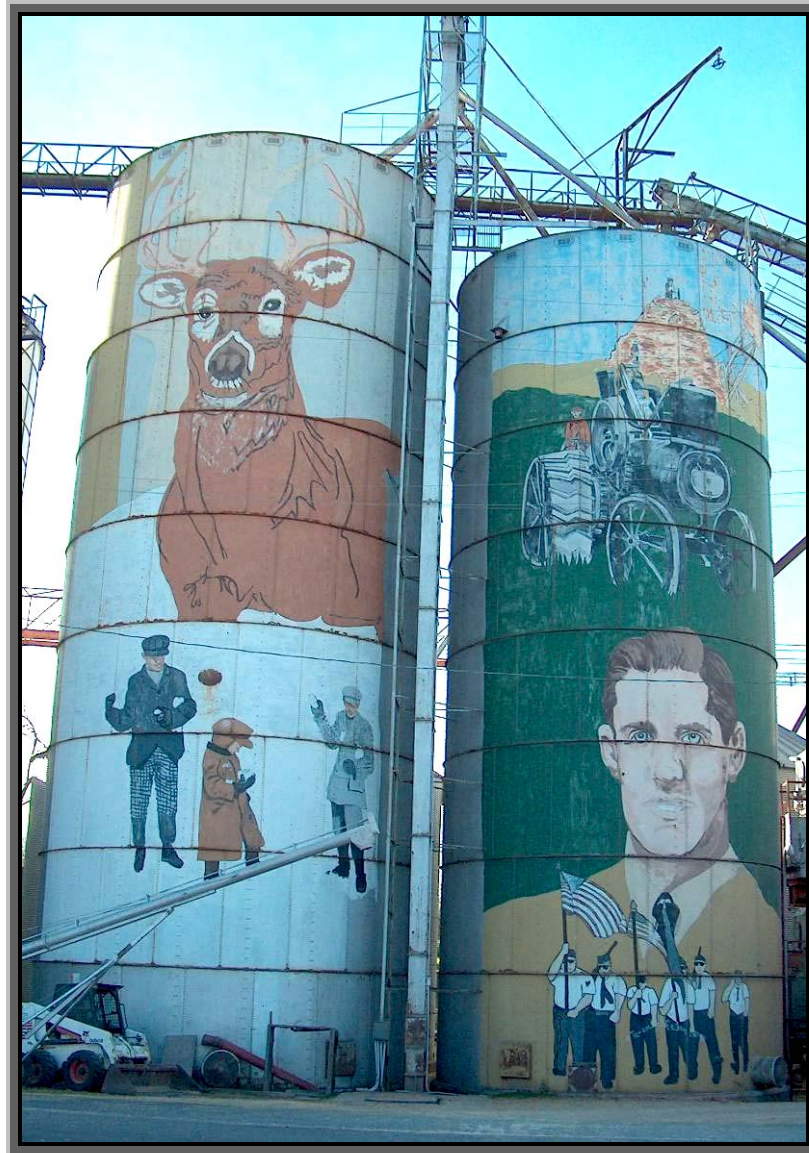
Figure 66: Detail of storage silo murals
