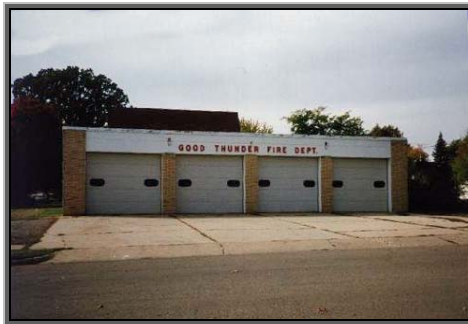
Figure 61: Good Thunder Fire Station, 1965 (Photograph courtesy of Sara Froehlich)
