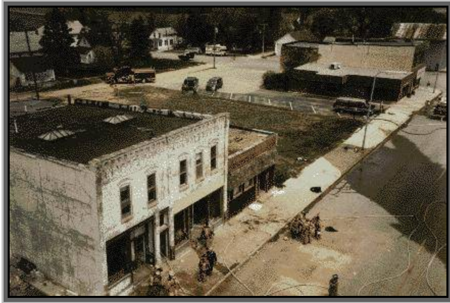
Figure 85: Condemned buildings on Main Street, 1993 (Photograph courtesy of Sara Froehlich)
