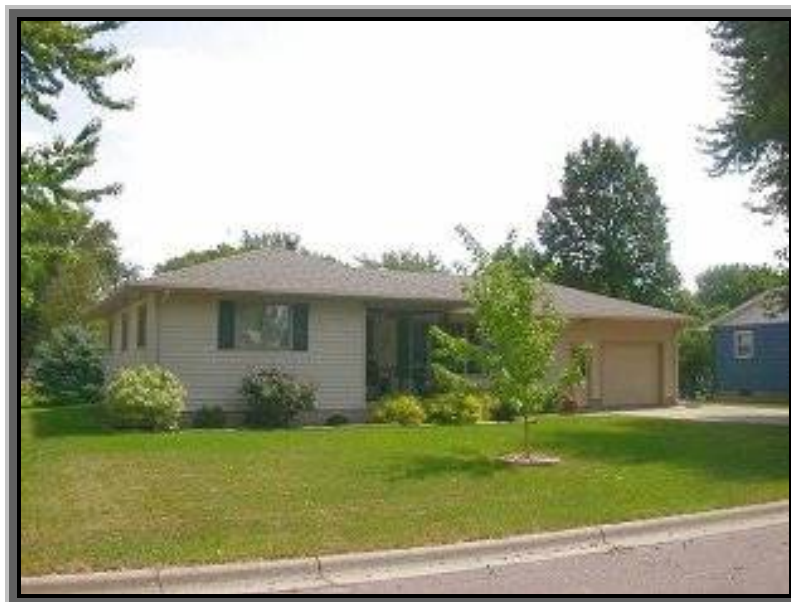
Figure 60: 129 Middle Street, built in 1974 Minimal traditional architecture. (Photograph from the Blue Earth County Assessor Office [online database])
