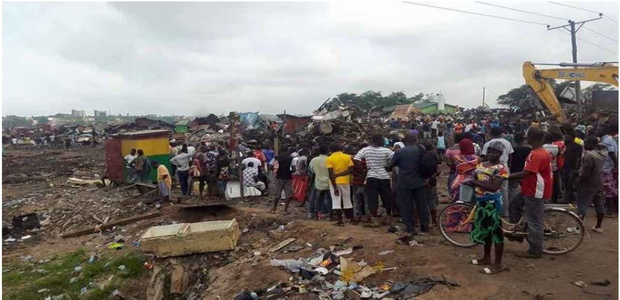
Figure 2: Demolition of Parts of Sodom and Gomorrah
