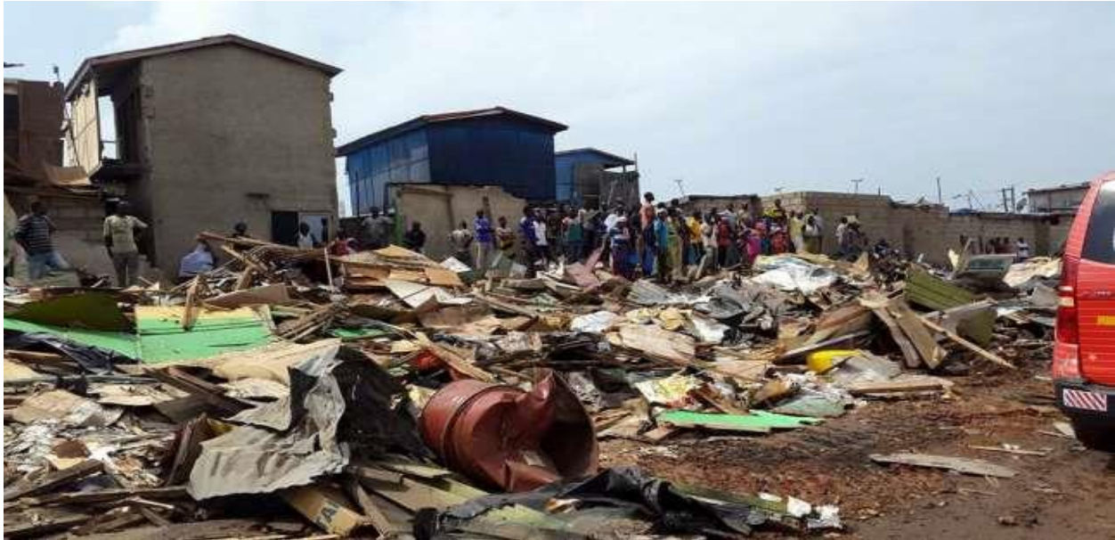
Figure 7: Aftermath of Demolition
