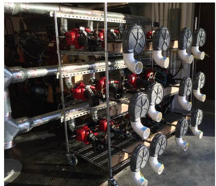
Figure 7-All 12 trimmers in two cycle mounted to aging rack
