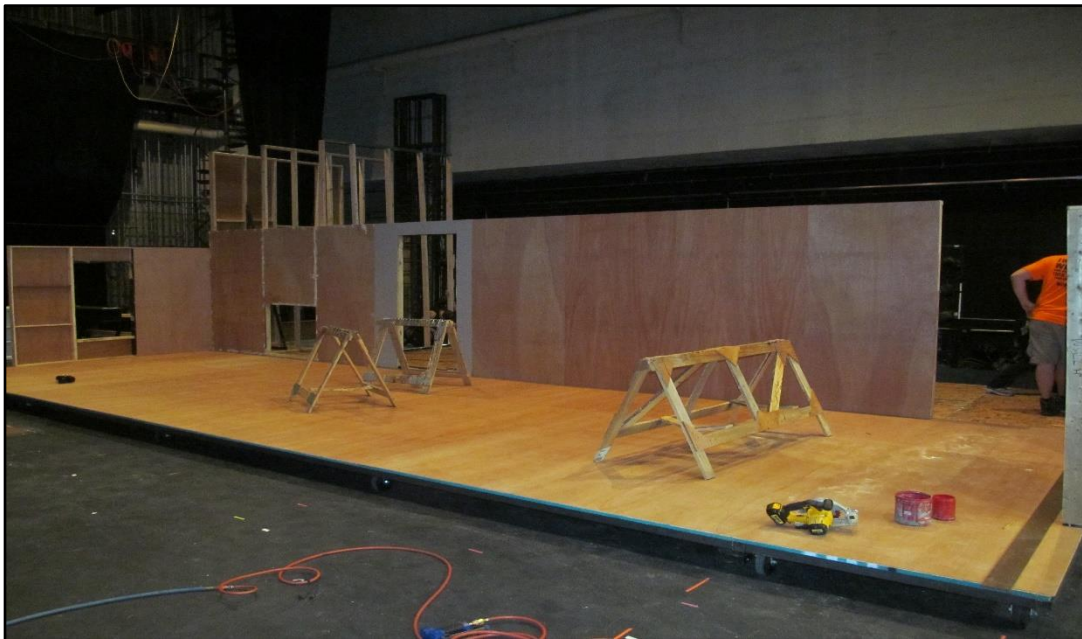
LAUAN LAID IN ACTING AREA. FIRST FLOOR WALLS INSTALLED.
