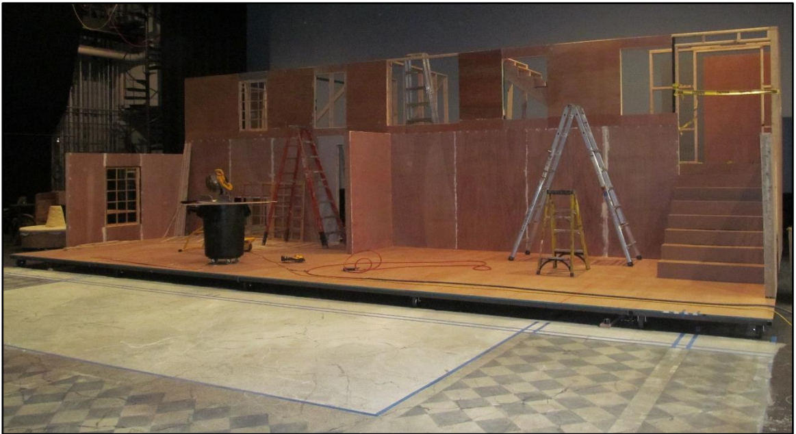
ALL STUD WALLS ARE UP. SECOND FLOOR ESCAPE STAIRS INSTALLED.
