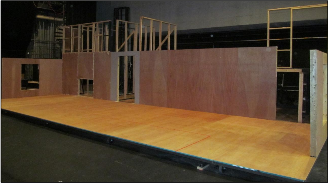
SOME OF THE ATTIC STUD WALLS INSTALLED.
