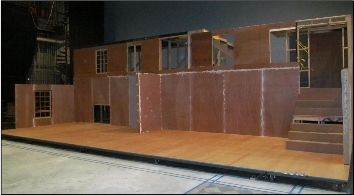
END OF DAY 3. PLATFORMS FOR ATTIC NEARLY COMPLETED.
