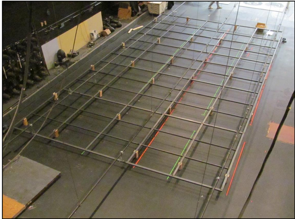
COMPLETED FRAME ON BLOCKS IN PREPARATION FOR CASTERS
