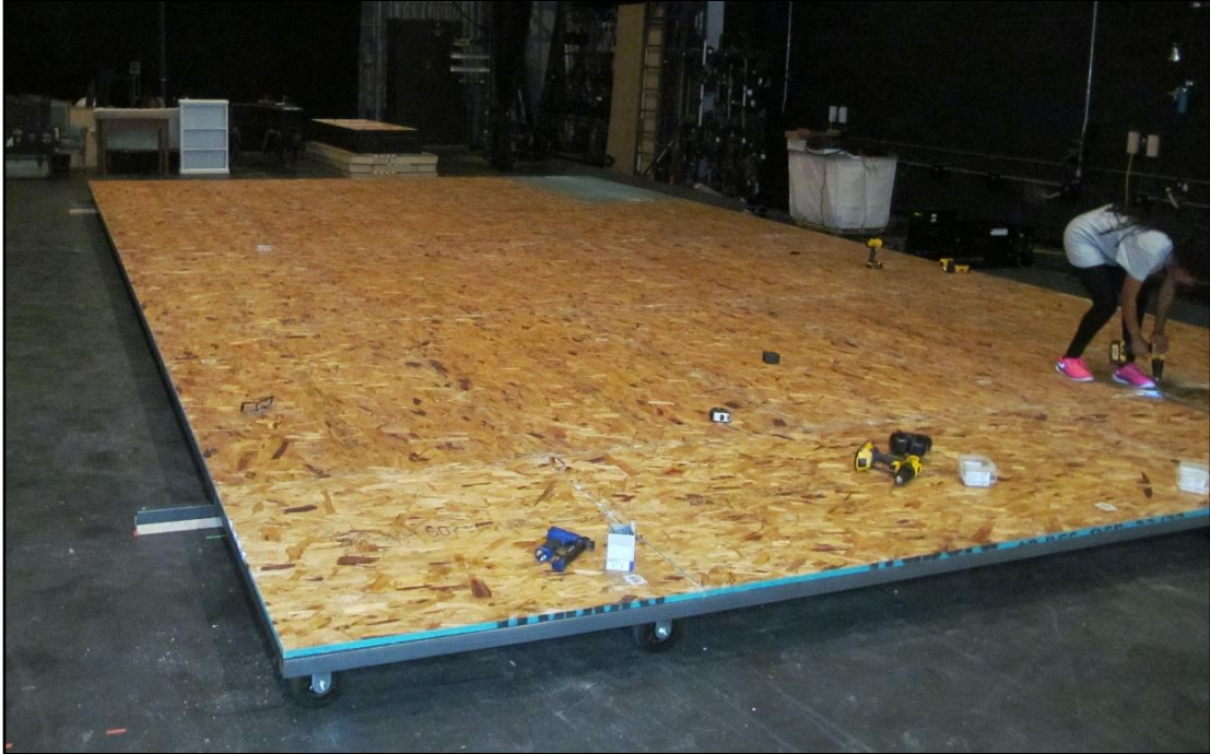
LAYER OF 3/4" OSB INSTALLED
