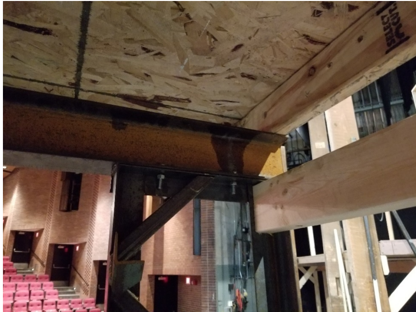
INSTALLATION OF I-BEAM ON 'STAGE UNIT'
